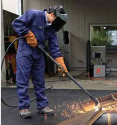
Cut with added reach
